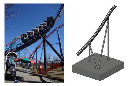
pairing the measurements taken from the sensors and gages with the data collected from the 3D scanning, we are breaking through that barrier to reach the cutting edge of technology. That allows for the section as a whole to be completely verified and accurately monitored moving forward. The ECM model provides a realistic sense of the as-built structure, and not what the design "should" have been.
