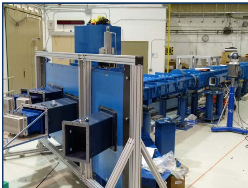
Figure 11 – Assembled Reactor Hall Vacuum Vessels with Wall Penetration Plate
